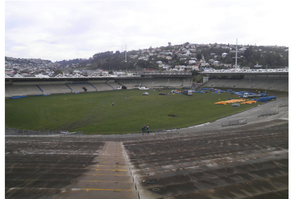
17 Photo of Carisbrook stadium during demolition
